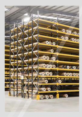
an adjustable pallet racking system creating the depth required to store long rolls. The beams for carpet racking can be decked in a choice of suitable materials including steel, chipboard, MDF, and open / close boarded timber. On this installation the timber was faced with a foam and timber chocks at each end to offer extra support.
