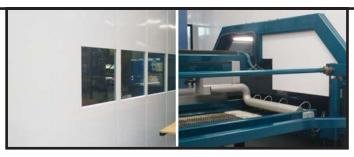
capping was utilised for lineal stability with additional strength coming from inline 50mm x 50mm RHS mullions fixed to the floor with countersunk M10 expansion bolts through 200mm baseplate.
