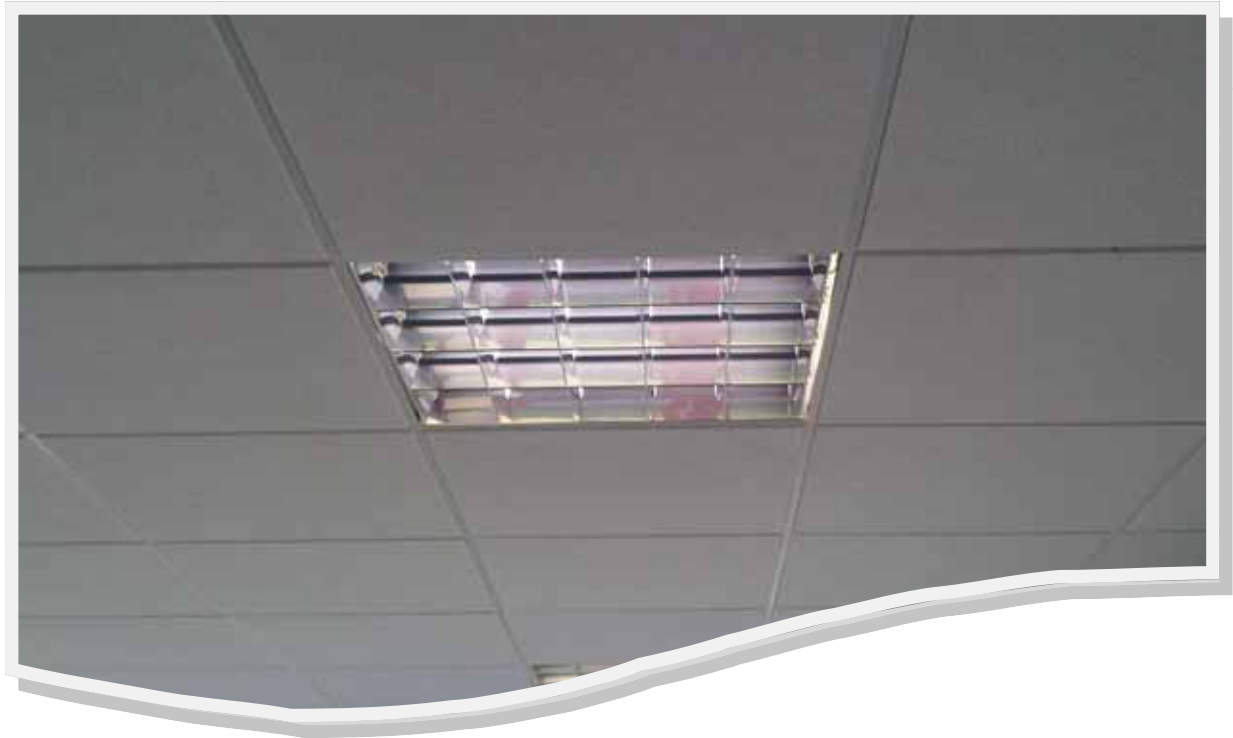
For Ceiling spans of up to 4800 mm, Beam & Lee Grid Suspended ceiling
