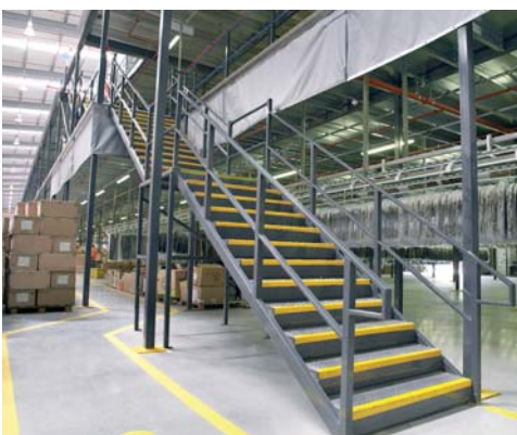
Part M Staircase
